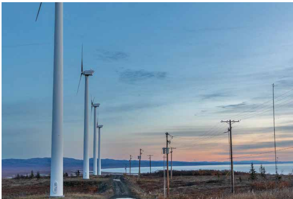
Photo by Werner Slocum, NREL 74116
